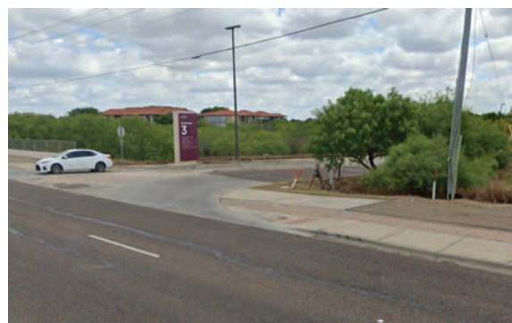
Bicycle Facility along Bob Bullock Loop
