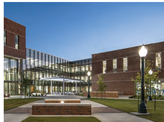
Light fixtures at connector, Tarleton State University, Applied Sciences. Photo credit: Coleman & Associates
